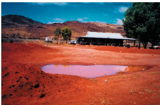
In this picture storm water which has fallen on the roof of the house and the surrounding compacted open areas and roads has collected in the mound. There are a number of ways of collecting storm water and mound systems are one of them.
