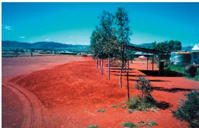
To improve the situation in the above picture, the compacted surface needs to be repaired so it can collect and absorb storm water before it causes erosion.
